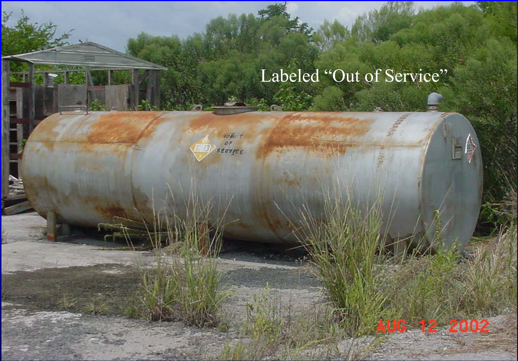
“Permanently closed” aboveground storage tank
